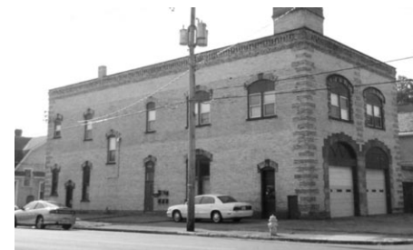
Hilltop Fire Station
